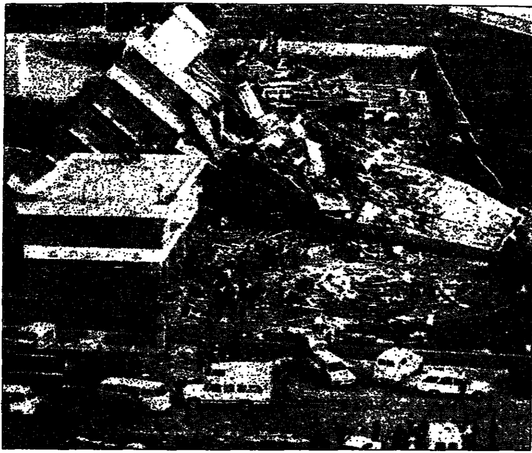
The Iraqi Embassy in Beirut after the bombing Tuesday, which caused the building to collapse.
